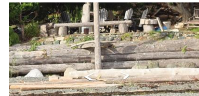
Figure 8 An example of a retaining wall/bulkhead made with logs. RC4S Imagery, Mitch Miller.
