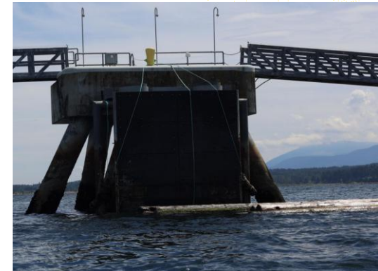
Figure 49 - An industrial overwater structure. RC4S Imagery, Mitch Miller.
