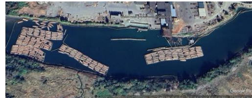
Figure 41 Vertical pilings secured with horizontal logs to hold/corral processed logs. Image © 2025 Airbus via Google Earth Imagery Date: 10/10/2022.
