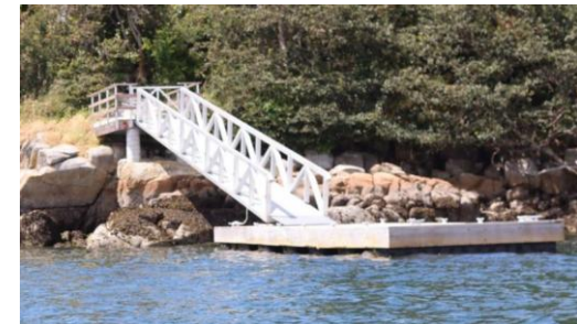
Figure 58 – A floating dock with a ramp/walkway linking it to the shoreline. RC4S Imagery, Mitch Miller
